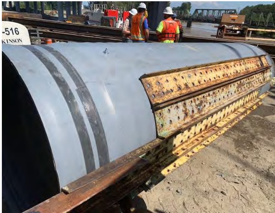
Figure 5: Confined Bubble Curtain Used at Tacoma HOV Project.
