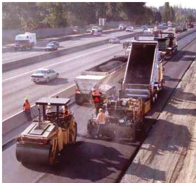
Construction crews adding lanes to I-405.
