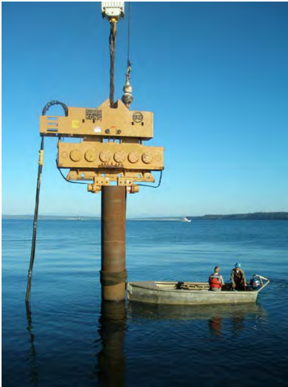
Figure 7. Driving complete on 36" pile.
