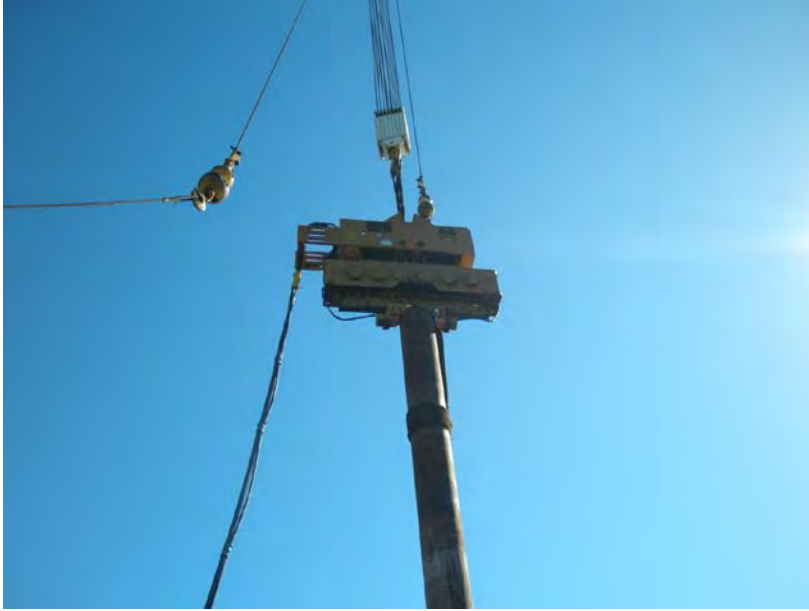
Figure 6. Driving 30" pile.
