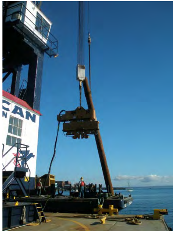
Figure 5. Crane pickup up hammer and 30" pile.
