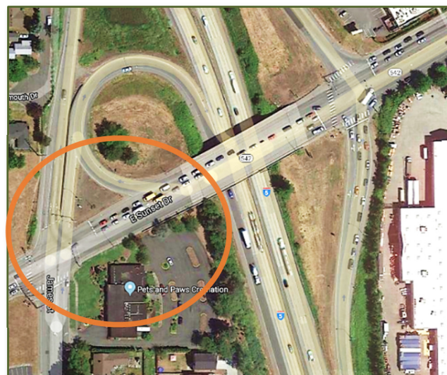
Exhibit 6-3: SB on and off-ramp at I-5 / E. Sunset Drive.
