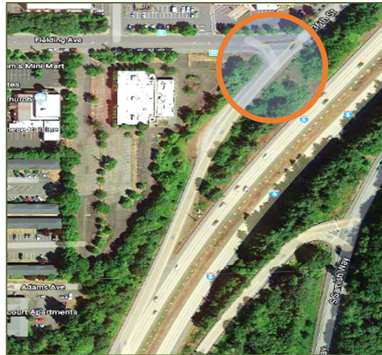
Exhibit 6-6: SB on-ramp at Fielding / 36th Street to I-5.
