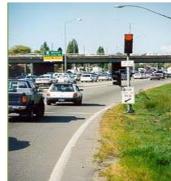
Ramp meter on I-5 in Seattle.
