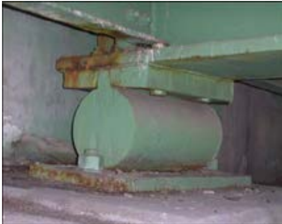
Figure 146. Surface rust on moveable bearing.
