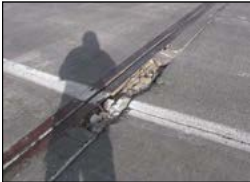
Figure 148. Spall in joint header. (Source: Colorado DOT)
