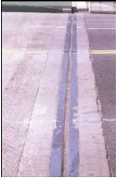
Figure 147. Joint partially filled with debris.
