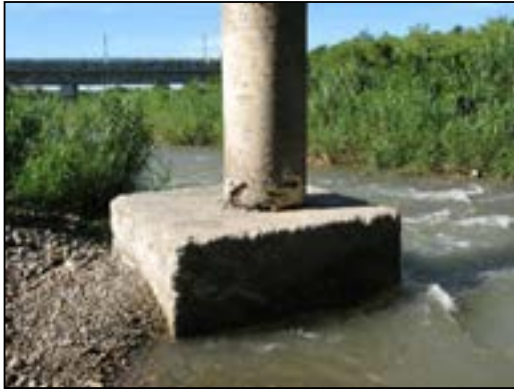
Figure 153. Exposed column footing in stream.
