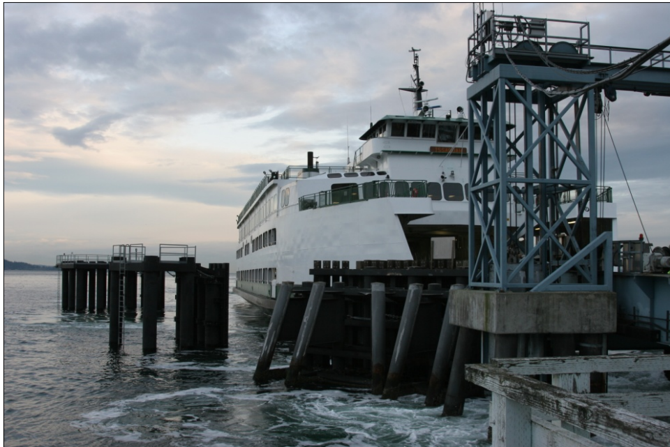
Vashon Ferry Terminal Slip 1 Exhibit 330-1
