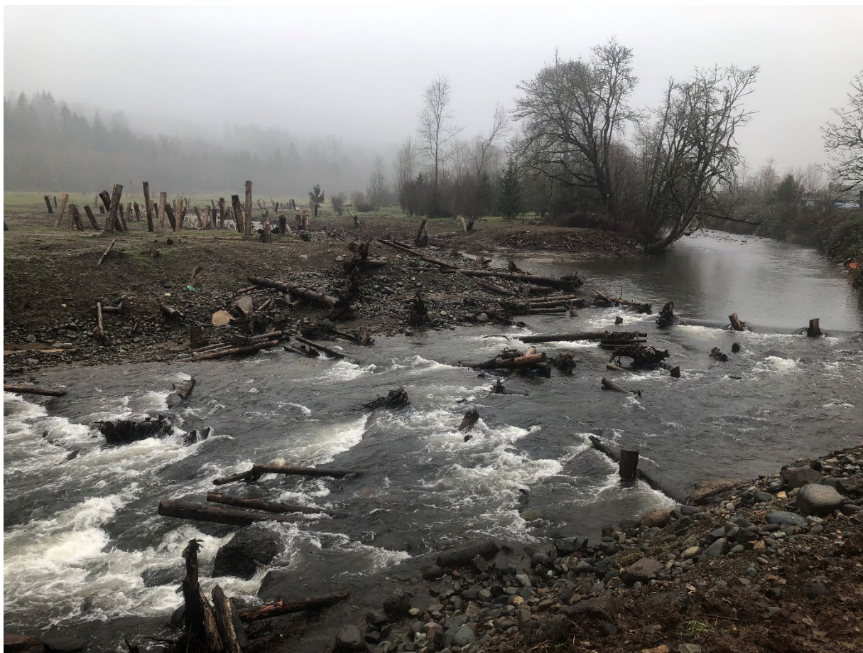
Figure 10-8 Example of Large-Channel Wood Grade Control
