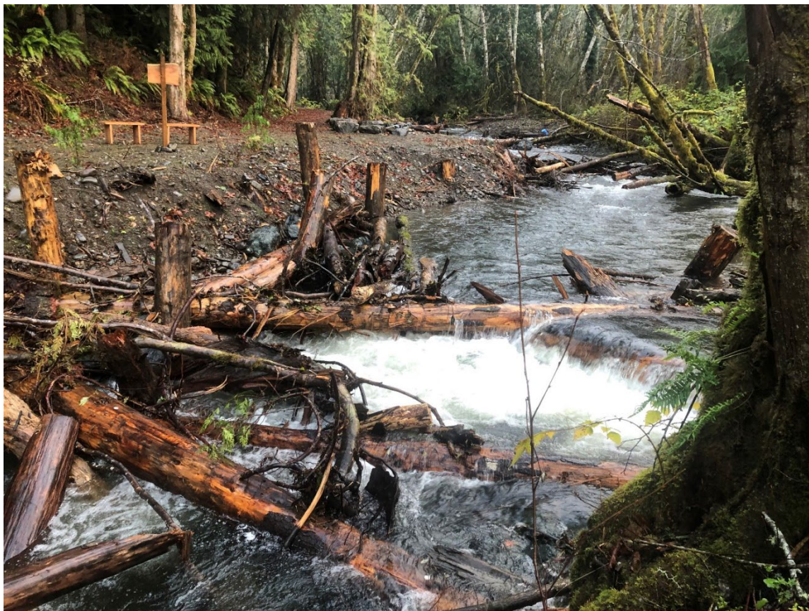
Figure 10-6 Example of Small-Channel Complex Log Grade Control
