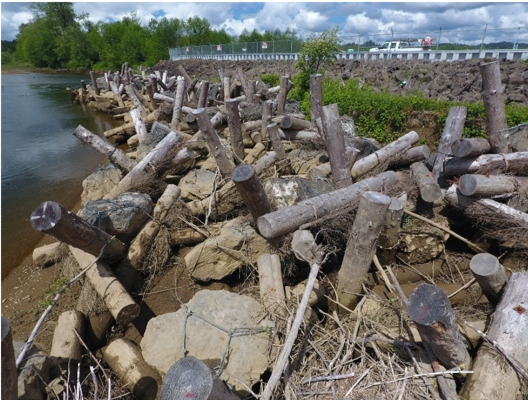
Figure 10A-10 Log Jacks, Wynoochee River, Grays Harbor County
