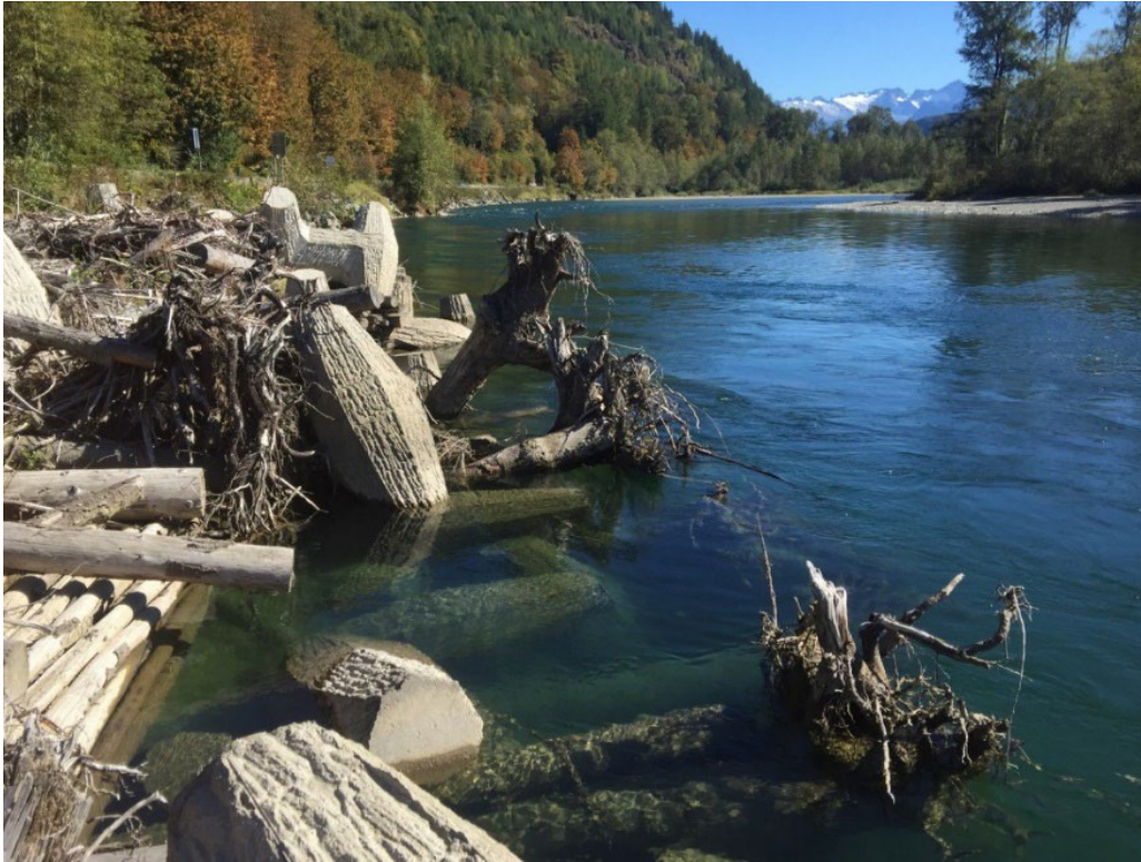
Figure 10A-9 Dolotimber Structures, Skagit River, Skagit County
