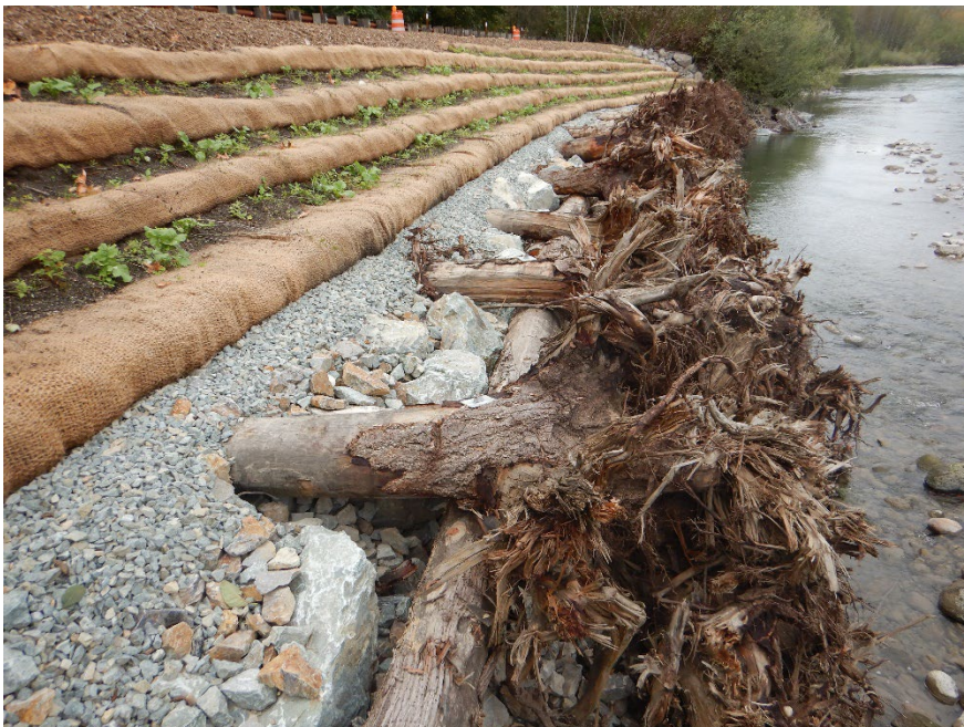
Figure 10A-6 Crib Wall with Soil Lifts (No Piles), Sauk River, Skagit County
