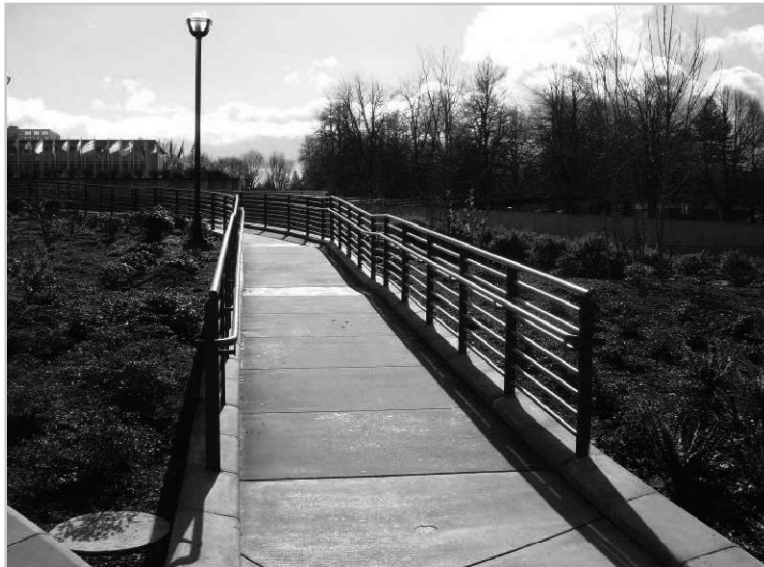
Access Ramp With Accessible Handrails
