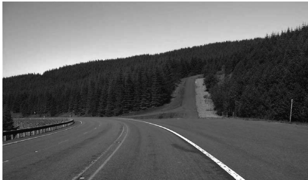
Emergency Escape Ramp Example Exhibit 1270-10
