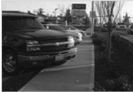
This Exhibit depicts a condition where the PAR has been reduced to less than the minimum clear width, resulting in an unacceptable condition.
